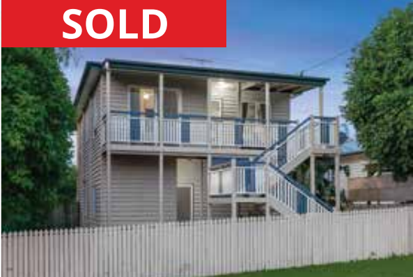
51 Faine Street Manly West
