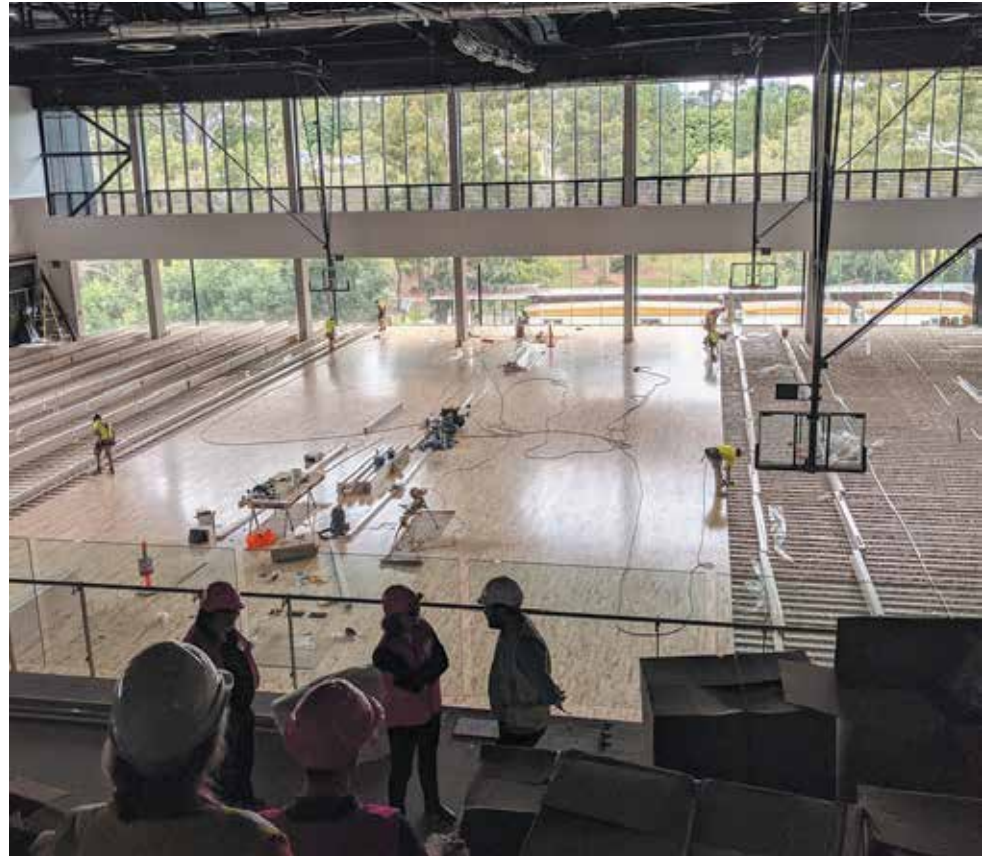
Iona College's Provence Centre is nearing completion. Photo: Supplied.
