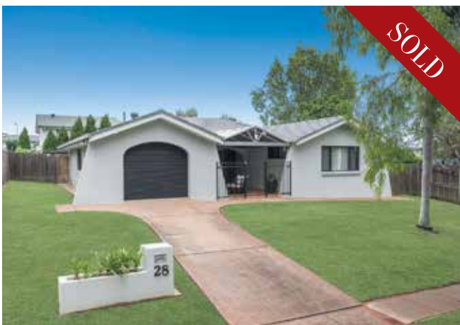
28 BARRAMUNDI STREET, MANLY WEST
