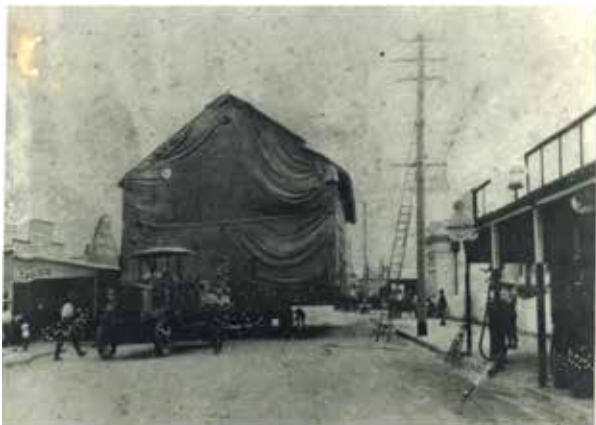
Journey of church along Edith Street, 1930. Electricity wires stretching across the street had to be disconnected, to allow for the height of the building.
