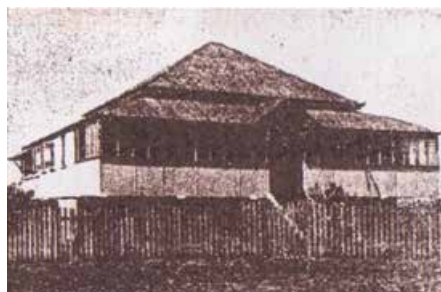
Original Farmhouse (Friary) in 1953 at Wynnum North.
