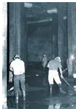
Cleaning out Roles Hill No. 1 Reservoir in 1969.
