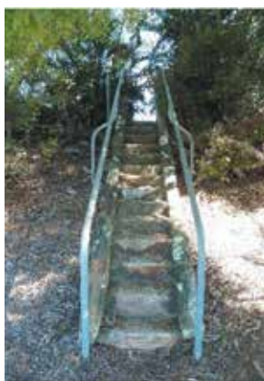
Steps from Preston Road to top of Roles Hill No. 1 Reservoir.
