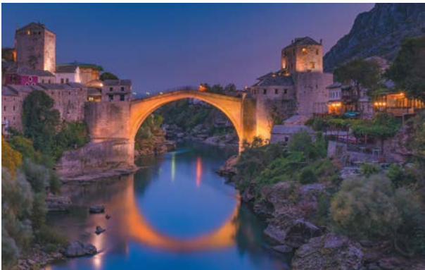
Mostar Bridge by Valerie Kleindienst
