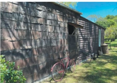
Rear Wall showing flattened kero tins.
